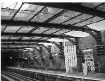
Compression struts requiring strengthening
